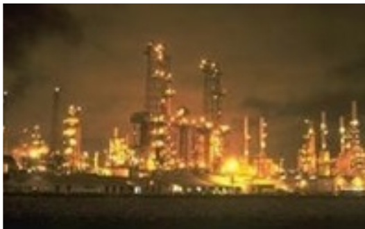
Chemicals Ex: 0,067 t/ton Aniline Petroleum refining (desulphuration & hydrocracking) 10-100 km 3 /h
